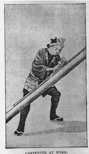
Carpenter at work. 仕事中の大工
