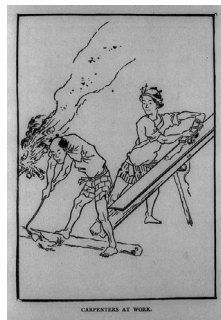
Carpenters at work. 大工仕事
