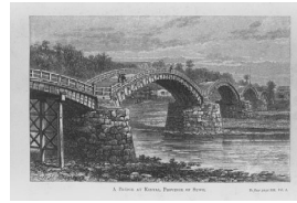
A Bridge at Kintai, province of Suwo. 錦帯橋, 周防地方
