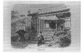
A guard house. 衛兵所
