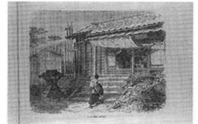
A guard house. 衛兵所
