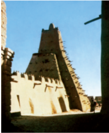
Fig. 7 Frank Willett, op. cit., p. 126. This mosque of the 14th century in Timbuktu is another proof of how Africans could adapt styles to their environment.
