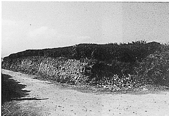
Fig. 5. A rammed bank supposed to be a rampart of the Liangchu period.
