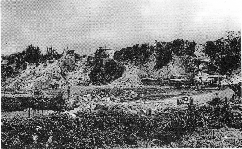
Fig. 1. The outer walls of Shurijō after its pulverization, May 1945.
