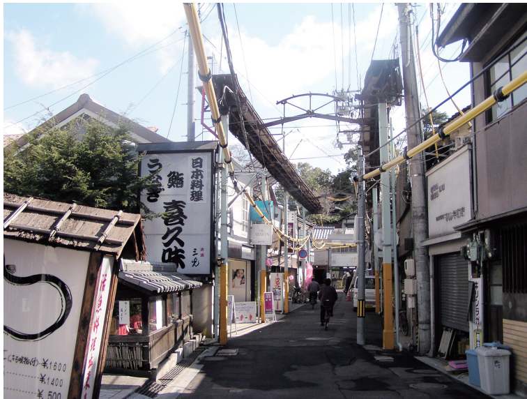
photo 4. Tearing down a Section of the Arcade in Kurashiki
