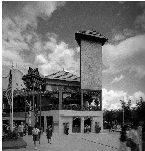
Figure 8. Philippine Pavilion at the 1992 Universal Exposition at Seville, Spain; designed by Francisco Mañosa,. Source: Raul Cesar Alonso de los Rios Rispa and Maria Jose Aguaza, eds., Expo '92 Seville: Architecture and Design , Milan and New York: Electa and Abberville, 1993.
