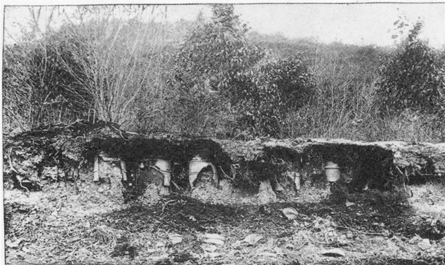
CYLINDERS in situ , KONABE.
